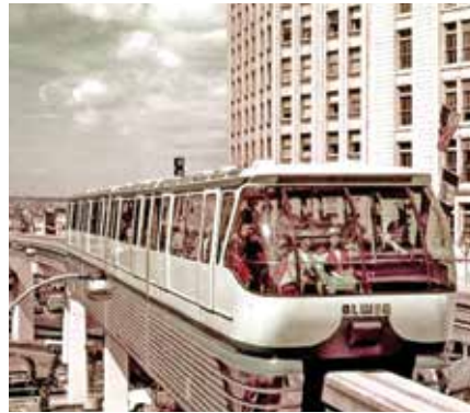
Figuras 3 e 4 - À esquerda Monotrilho Alweg Seattle ( https://www.seattlmonorail.com/about-the-monorail/ ) e, à direita, o sistema Safege proposto pela General Electric ( https://digitalcollections.lib.washington.edu/digital/collection/seattle/id/3584/ )
